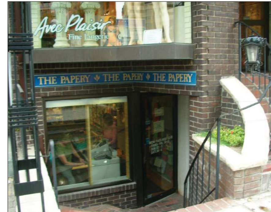
A split ground floor in Toronto, Canada has been opened up to create a store on the lower level.
